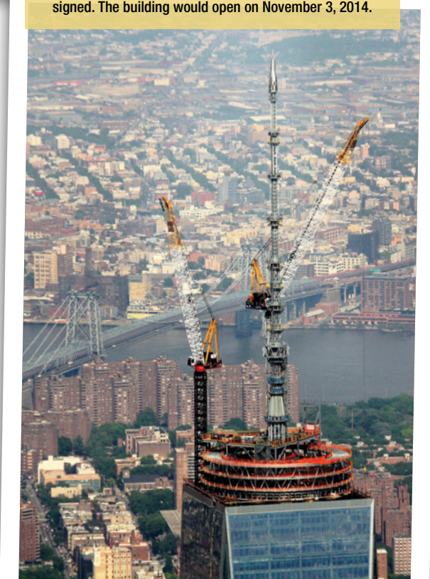
Cranes operated by Local 14 and Local 15 members place the final components of the spire at the top of the new One World Trade Center on May 10, 2013, making the structure a total height of 1,776 feet – a reference to the year in which the U.S. Declaration of Independence was signed. The building would open on November 3, 2014.
