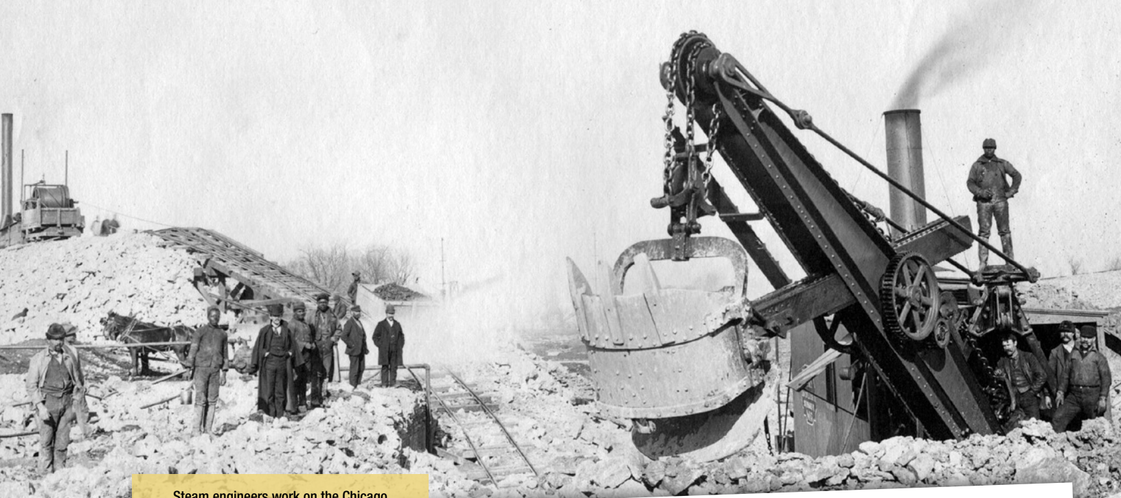
Steam engineers work on the Chicago Sanitary and Ship Canal in 1895, the year before the National Union of Steam Engineers (which would become the International Union of Operating Engineers) was formed. When it opened in 1900, the 28-mile canal project, the largest earth-moving operation in North America up to that time, connected Lake Michigan to the Des Plaines River and allowed for the reversal of the flow of the Chicago River. (Photos courtesy of the Chicago Metropolitan Water Reclamation District.)
