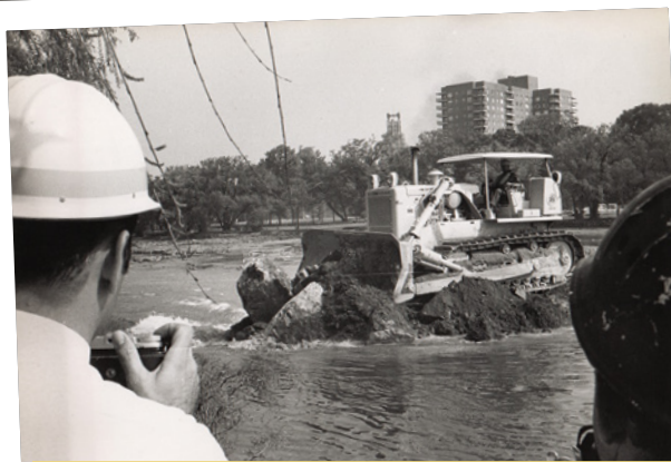
Members of I.U.O.E. Local No. 463 in Niagara Falls, New York, build the cofferdam that shut down the American Falls on the Niagara River in June 1969 for maintenance. (Photos courtesy of Niagara Falls Thunder Alley/www.niagarafrontier.com.)
